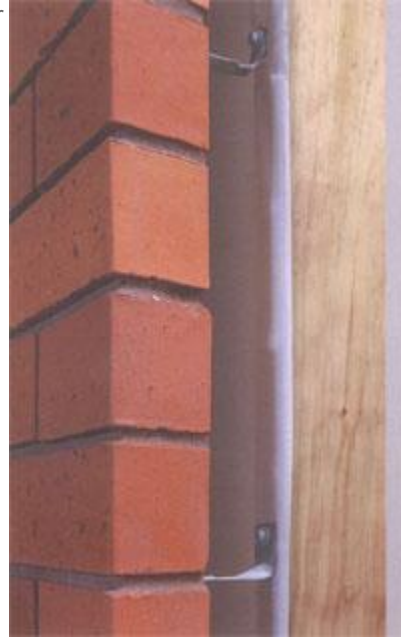
A wall detail showing the Monier Brickmaker's Cavity Brick system
